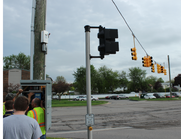
Figure 5: Intersection used for field tests. The targeted infrastructure controls a T intersection. The failsafe state of the intersection is a blinking yellow light on the main road and a blinking red light on the side road. At left is the traffic controller cabinet, which contains the controller, switch, and MMU. Radios and a video camera are located at the top of the pole.
