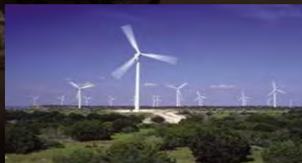
Power generation and distribution
