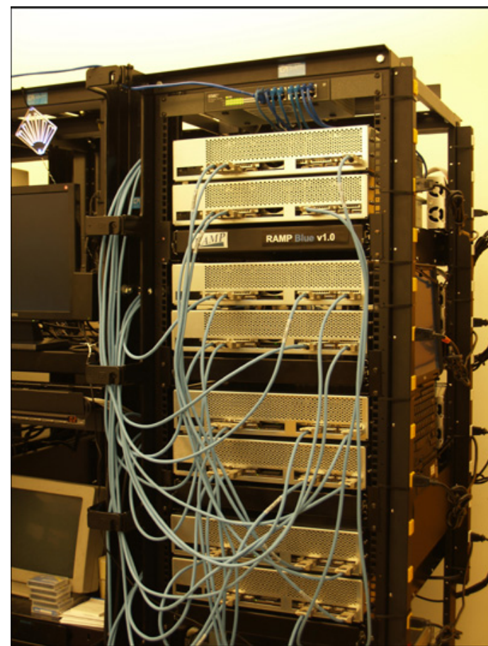
Ramp blue experimental platform, from the RAMP project.
