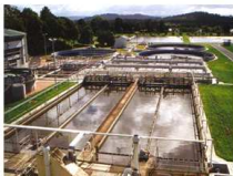
Sewage control system exploited by insider to cause sewage to flood the surroundings.
